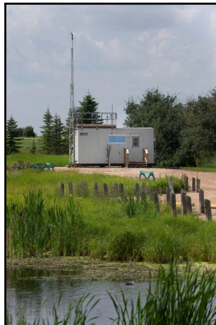
Figure SEQ Figure \* ARABIC 9: Range Road 220 Station
