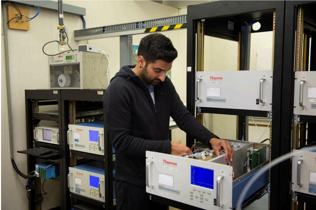
Figure 2: Continuous air monitoring station interior
